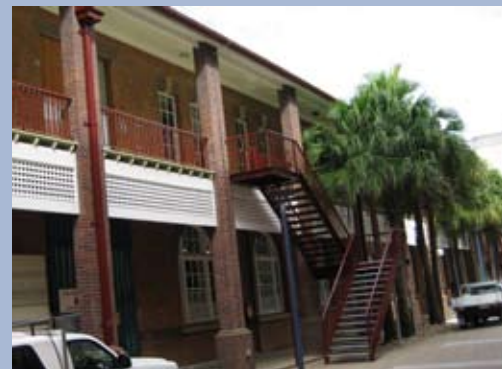
REPAINTING TO HERITAGE BUILDING, J BLOCK, GARDENS POINT.
